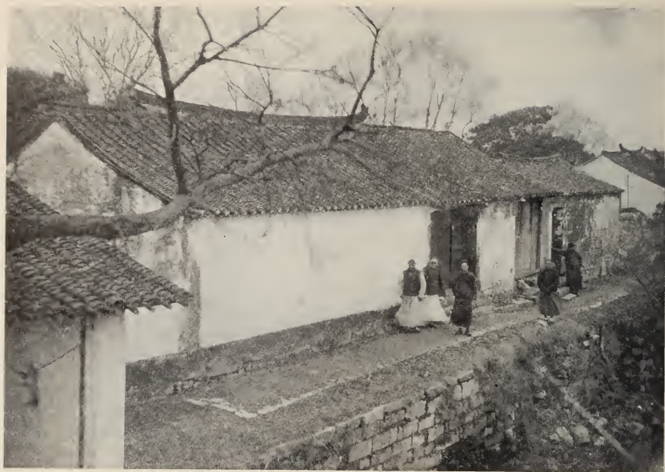
OUR NEW PROPERTY IN TAITSANG SEEN FROM THE CANAL
